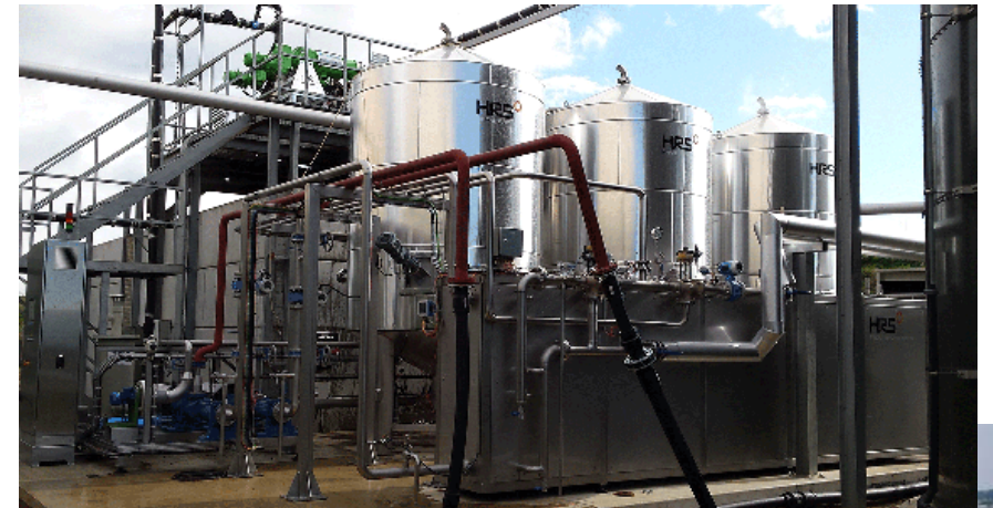
(a) Pasteurizers; (b) thermal hydrolyzers; and (c) macerator pumps
