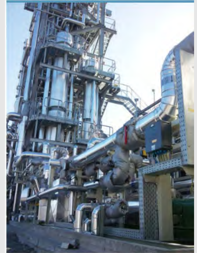
Gas Sweetening Plant
