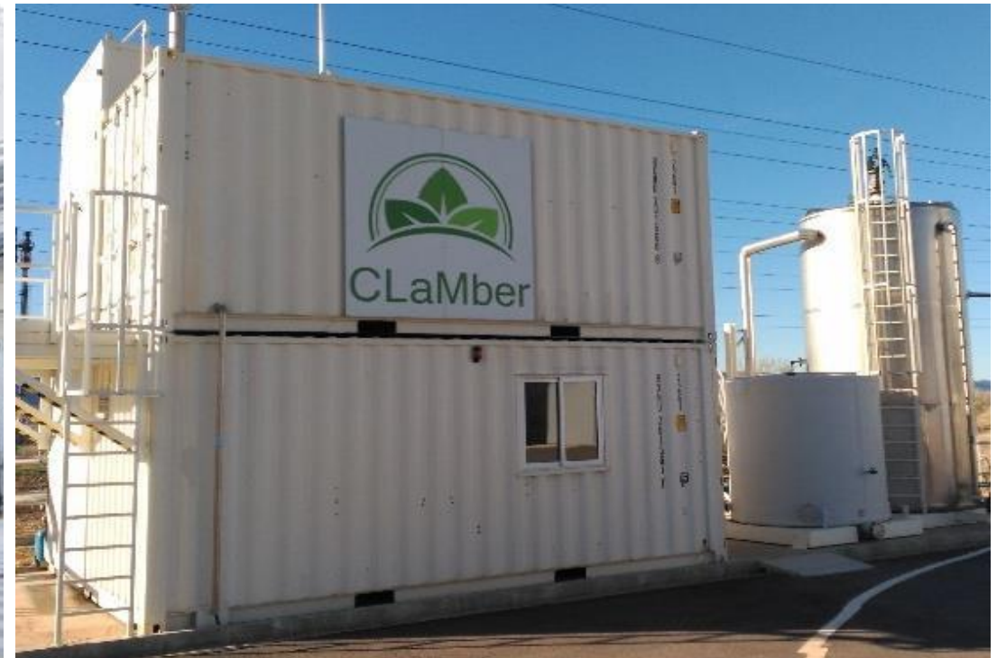
Industrial anaerobic digestion unit. CLaMber facilities (Puertollano, Spain)
